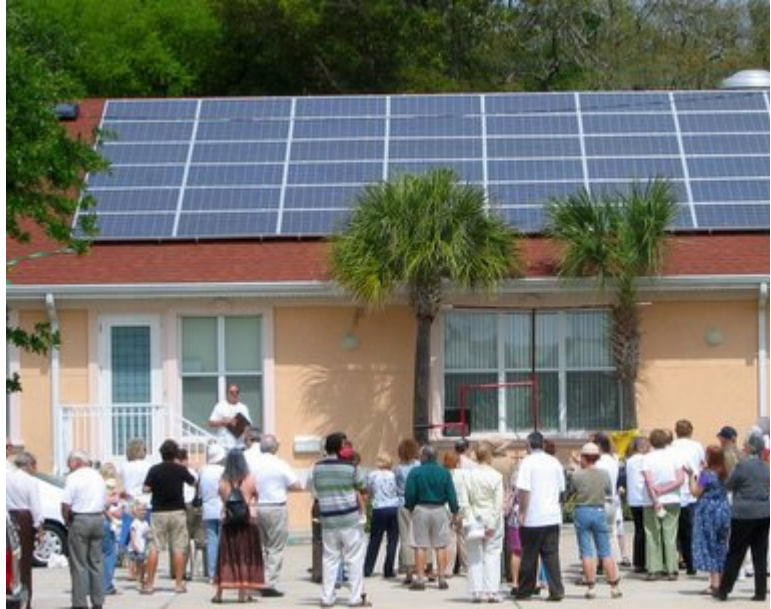
Solar panels added in 2008
